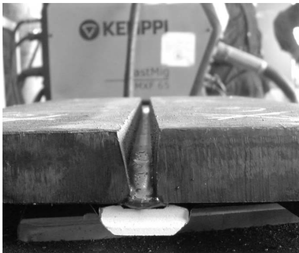
Figure 3. Joint 1 after the welding of root and first fill welds. Slika 3. Spoj 1 posle zavarivanja korenog i prvog zavara ispune
