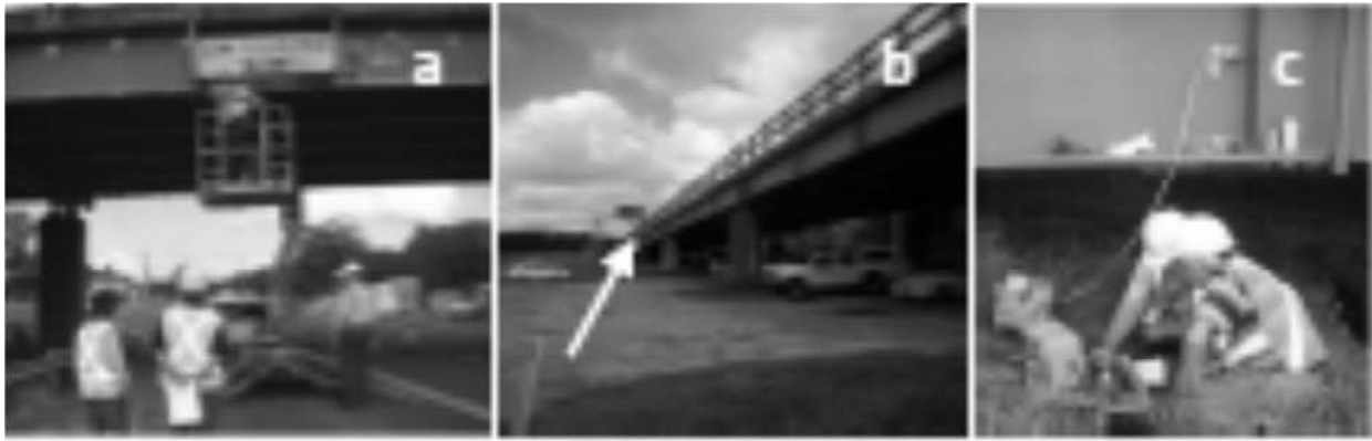
Fig. 5 Views of the steel bridge that was struck by a truck where the UltraMARS system was used for evaluation of the residual stresses.
