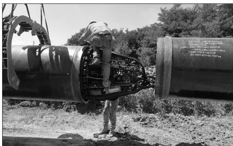
Figure 3. Internal centralizer IDC
