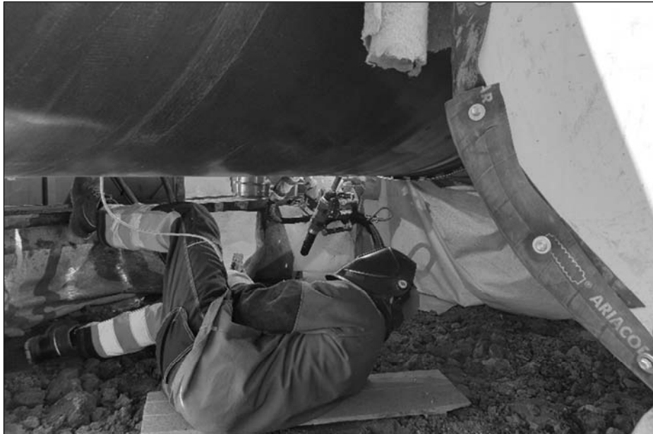
Figure 4. An Operator monitors the welding head operation in MAG process
