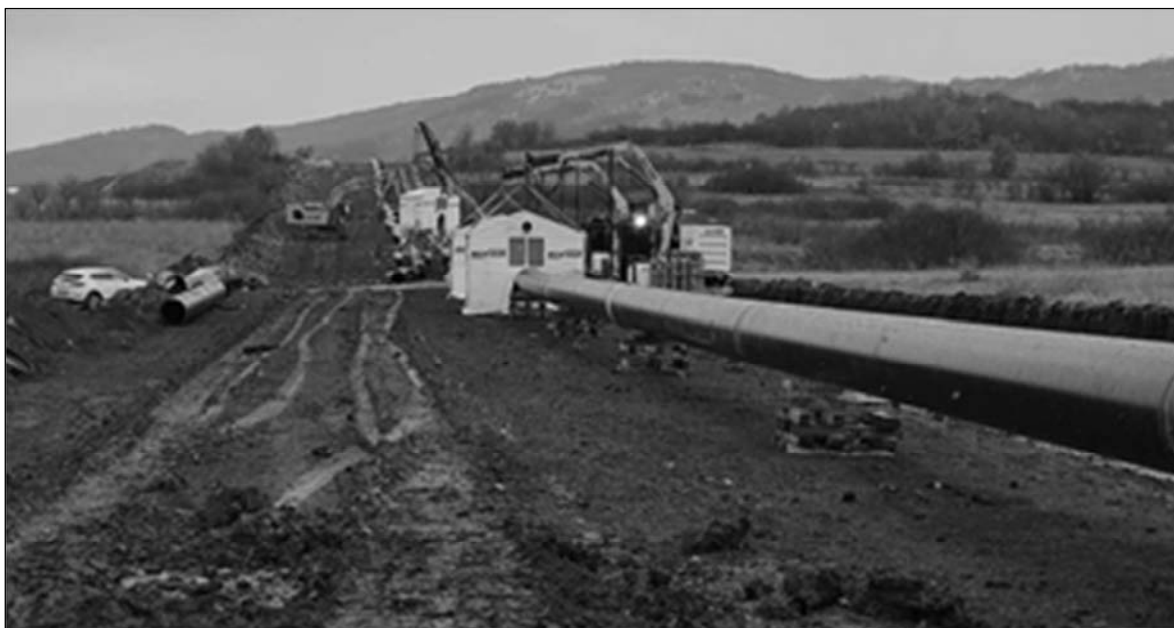
Figure 5. Welding on the route
